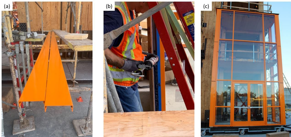
Figure 8: (a) Cover caps are installed after the pressure plates have been attached, (b) sealant finish is applied, (c) finished curtain wall
