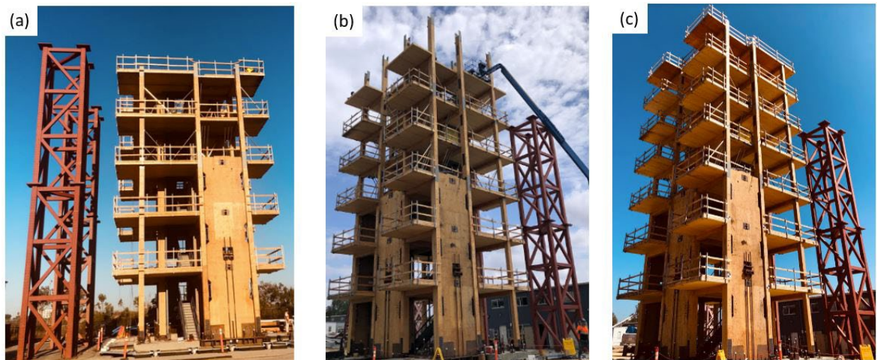
Figure 1: (a) Gravity framing complete to 5 stories, and the safety towers are installed, (b) erecting columns for the 6 th and 7 th stories, (c) gravity framing complete to 7 stories
